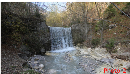
Main sediment storage dam
