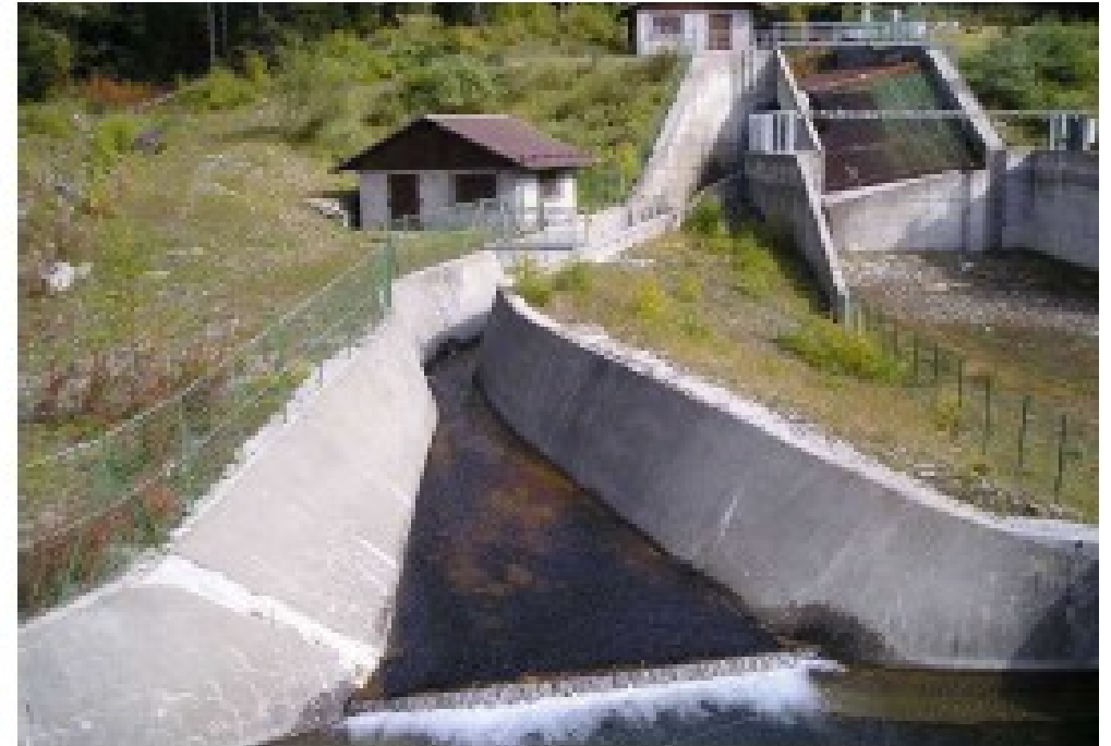
Figure 7. ARPAV monitoring station: frontal view of the depositional place and of the separating grid for the coarse bedload (from: Il Bacino Attrezzato del Rio Cordon, Regione Veneto, 1992), and outlet channel for the finer sediment deposition
