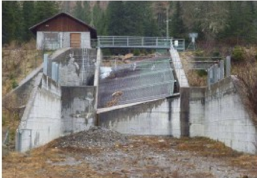
Figure 7. ARPAV monitoring station: frontal view of the depositional place and of the separating grid for the coarse bedload (from: Il Bacino Attrezzato del Rio Cordon, Regione Veneto, 1992), and outlet channel for the finer sediment deposition
