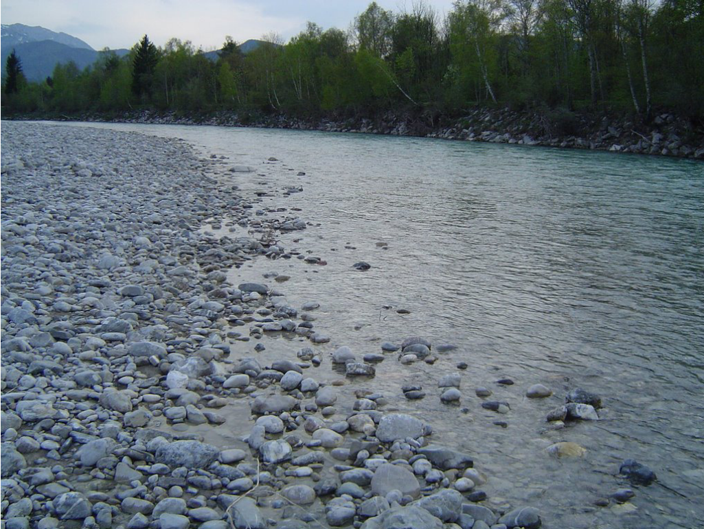
Figure 2: Bank obstruction and Isar near Bibermühle (Photo: panoramio.com – Gene666)
