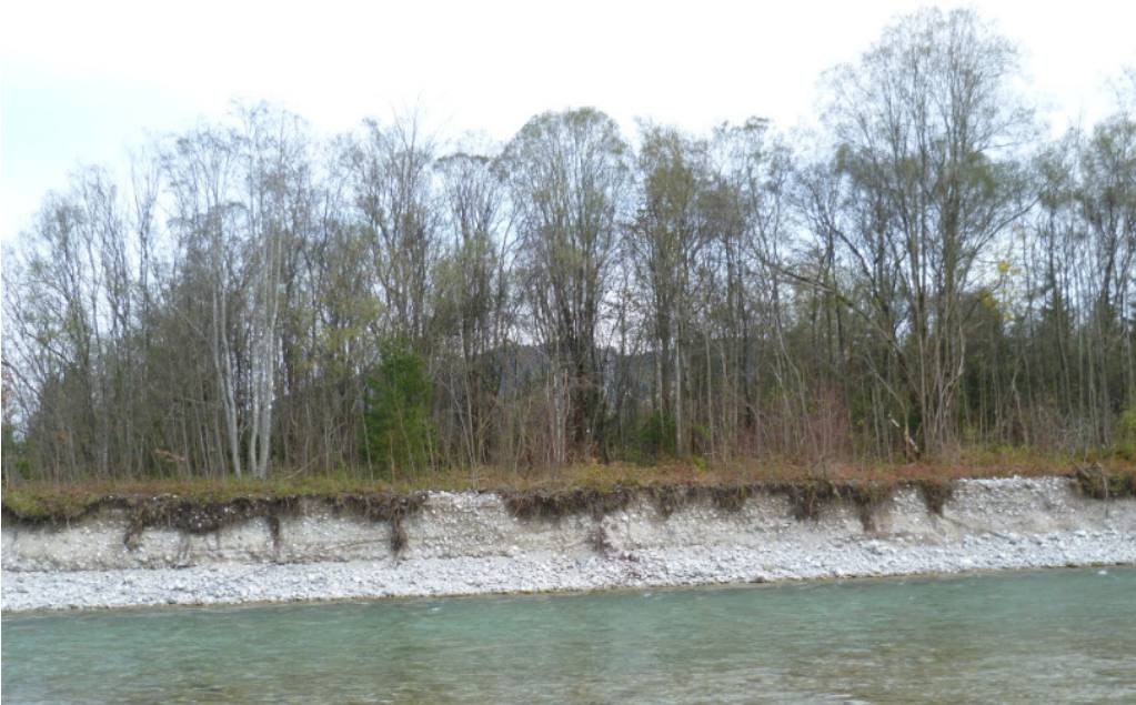
Figure 2: Erosion at the bank of the Isar near Arzbach mouth
