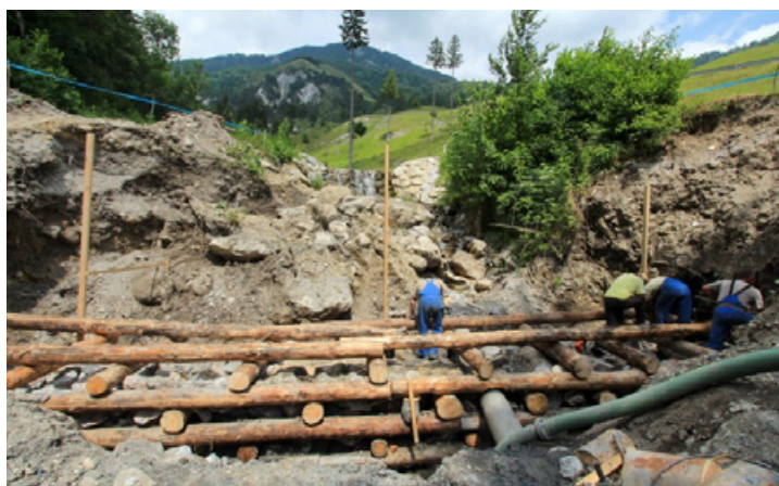
Figure 10 - 11 - Left: Wooden Cribwall on Pšatariver and right: building of wooden cribwall on Bistričica (13.06.2015).
