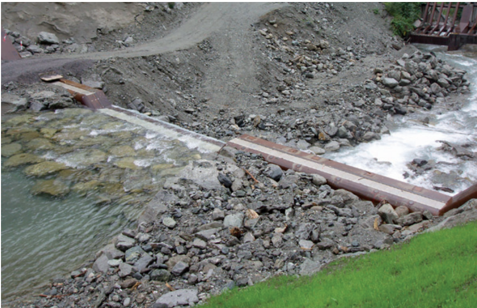
Figure 5 - Monitoring station at Suggadinbach torrent (Vorarlberg-Austria).
