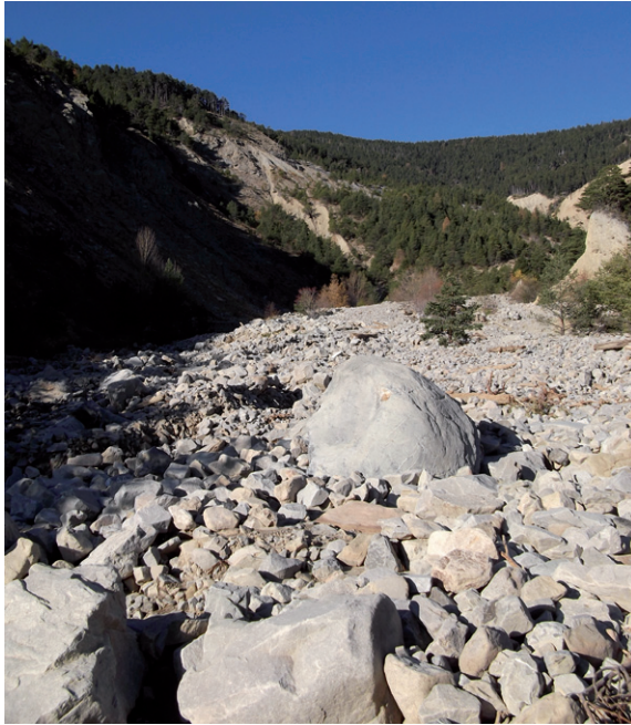
Figure 1 - Réal Torrent test bed in the Southern French Alps (Provence-Alpes-Côte-d'Azur Region)
