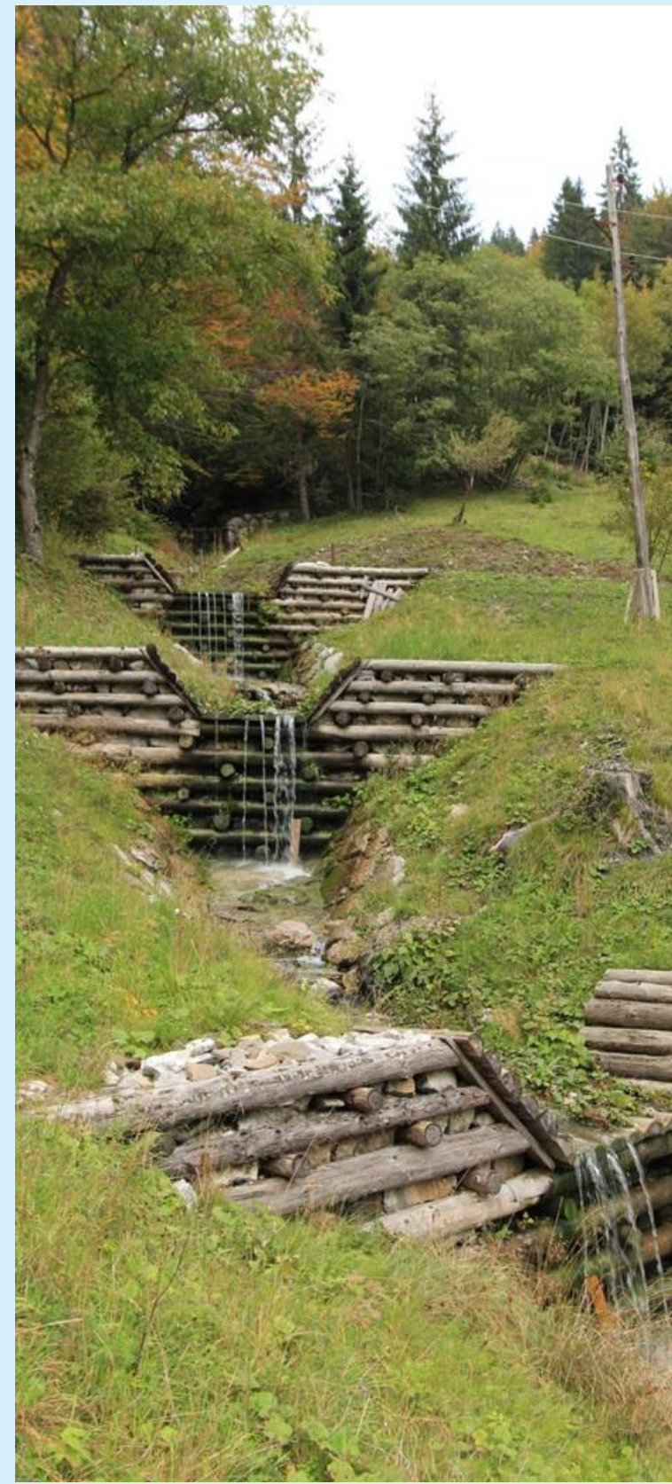
Figure 7: Cribwalls on the Torrent Čerinjščica
