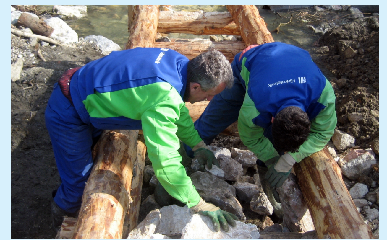
Figure 9: Building of wooden cribwall on the Pšata River
