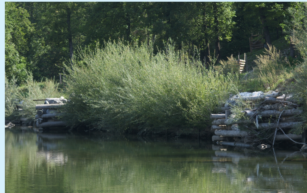
Figure 2: Wooden cribwall on the Savinja River
