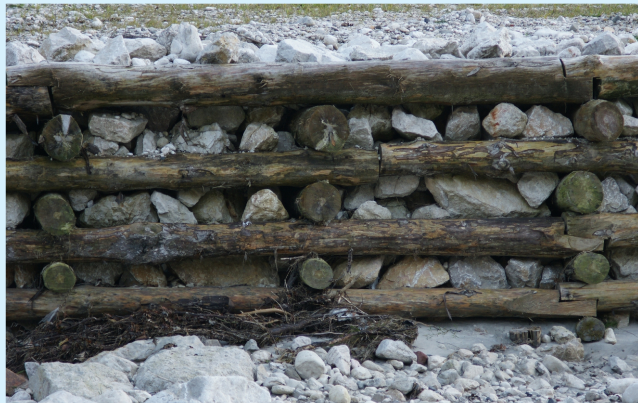
Figure 1: Wooden cribwall on the Sava Dolinka River
