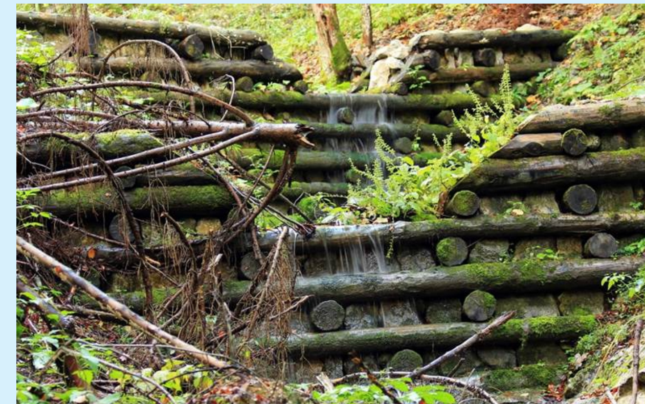
Figure 3: Wooden cribwall on the Torrent Kolovec
