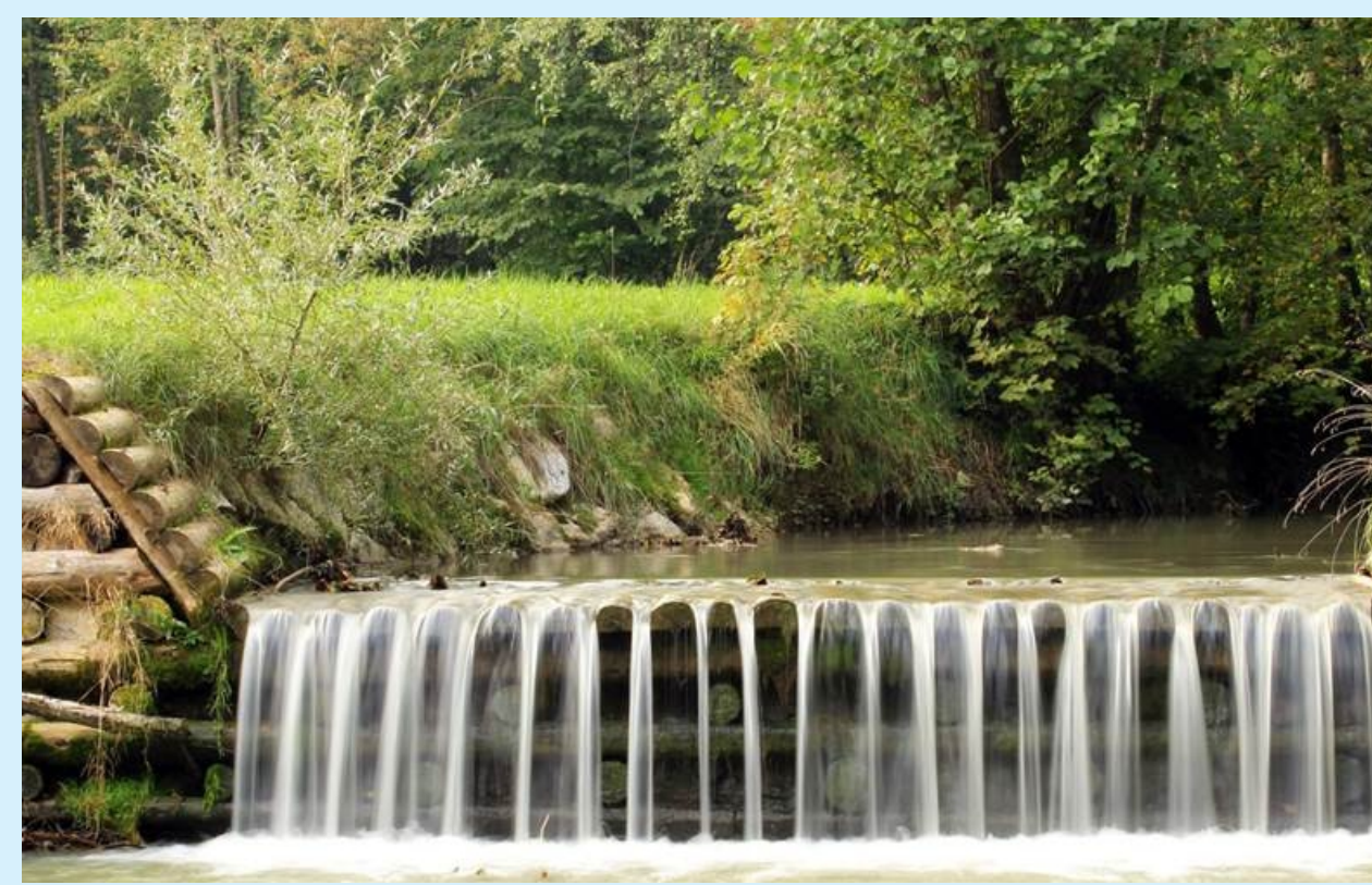
Figure 6: Wooden cribwall on the Pšata River
