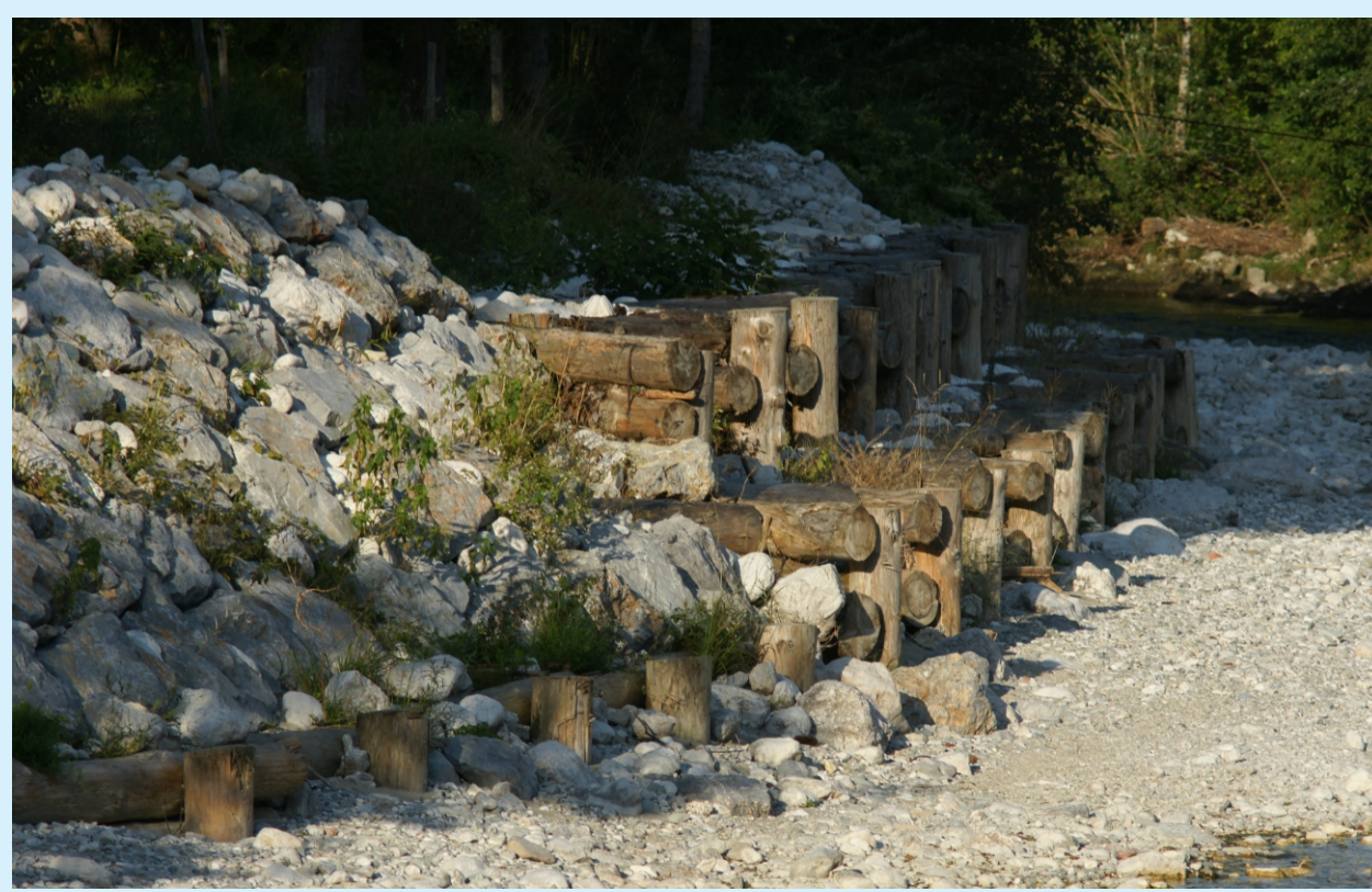
Figure 5: Wooden cribwall on the Sava Bohinjka River
