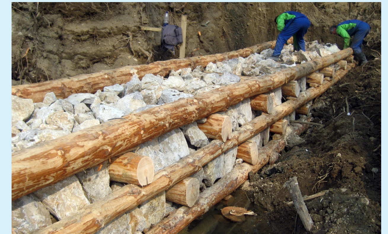
Figure 4: Building of wooden cribwall on the Pšata River
